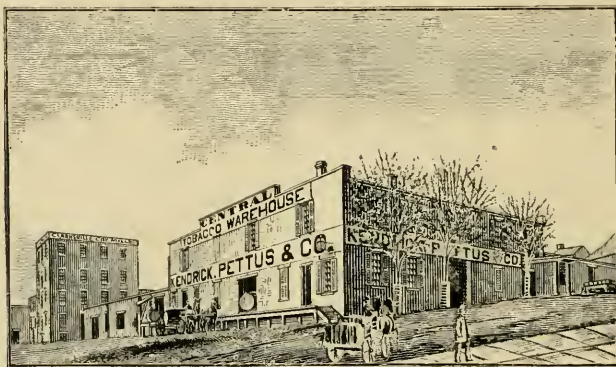
OLD CENTRAL WAREHOUSE.
